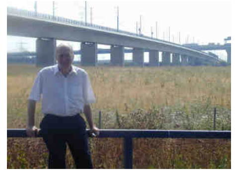
Andrew inspects the new Channel Tunnel rail link at Thurrock, to be opened in late 2007
